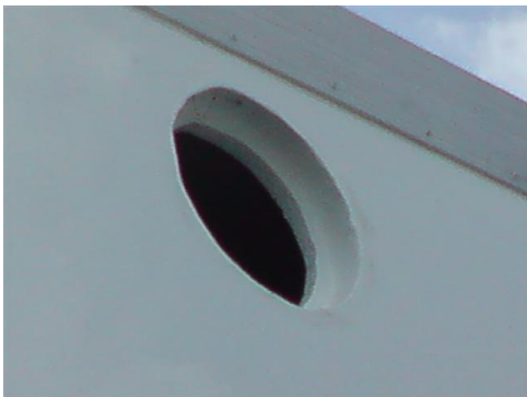
fan cut outs for flush mount extraction fans.
