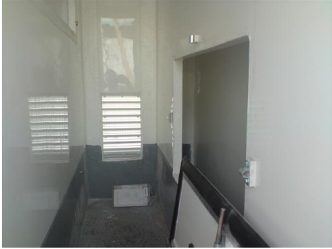
Service hatch removed to show false wall.
