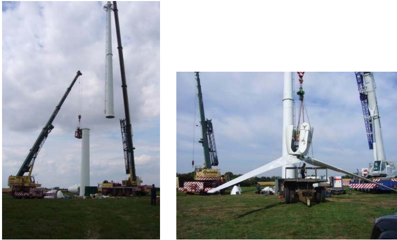
Photo 11+12 – Construction of Endurance turbine
